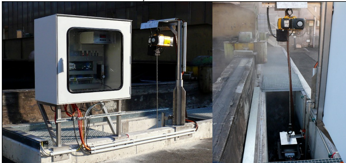
FLUCOmat with ultrasound controlled elevation system
